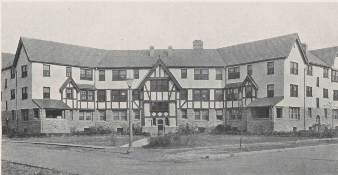
The Mackenzie Apartments, corner of Murray Avenue and Beech Street, Mariemont. This building, constructed of native quarry stone, stucco and half timber, with slate roof, contains nearly 30 apartments, each with three or four rooms and bath. Clinton Mackenzie, Architect, New York City
