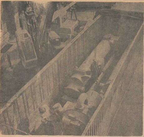
WORKMEN HAD THEIR hands full late Wednesday afternoon as they unloaded a giant compressor for the West Library's new air-conditioning system. After unloading it at the back of the Union Building, they were faced with the task of moving it into position through maintenance tunnels. When in place, it will help to cool the reference room, documents and maps department, technical processing department and the order department. Other rooms to be cooled include the third floor, largely taken up by the political science department.
