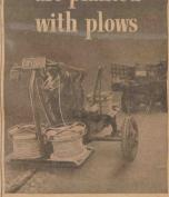
$\mathbf{R}^{\mathrm{URAL}}$  telephone wire—not in cables—can now go underground where bad weather and grass fires can't harm it.
